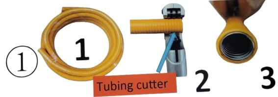
Use a tube cutter to remove 2 to 3 corrugations (waves) from the CSST tubing, ensuring the cut is smooth, flat, and free of burrs. **Do not** bend, twist, or flex the tubing to break it, as this can create significant burrs that may Damage the fittings and ultimately lead to a gas leak.
